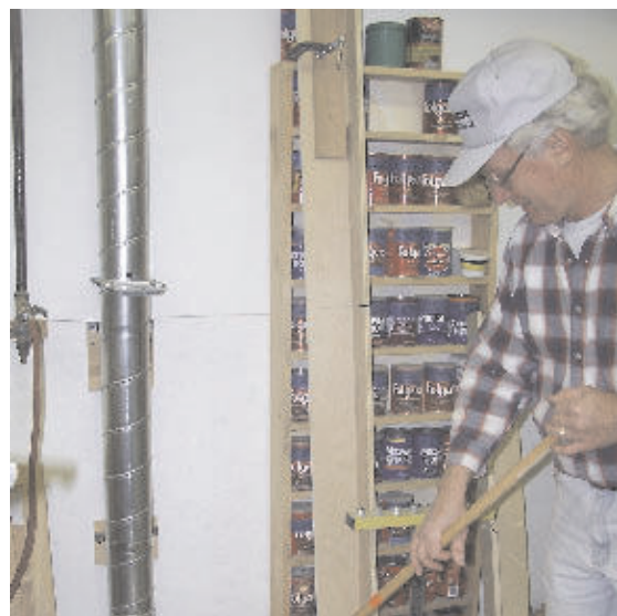
Return to come — Currently the new dust collection system at J&J Custom Woodwork in Stroudsburg, Pa., empties into a trailer outside. Plans call for finishing the system with a return air line so heating and air conditioning in the shop will function properly.
